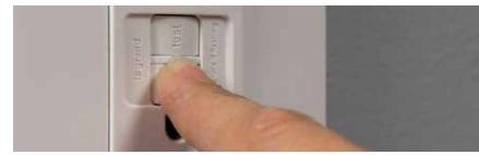
PREVENT IT Without a GFCI device that is accessible and easy to see, trips can easily go unnoticed, leading to much bigger problems. Power loss to sump pumps, freezers, or other important appliances can result in flooded basements or even more expensive property damage.
