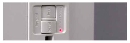
GFCI receptacles have a trip indicator light and test/reset easily with the push of a button. Breakers, however, can be confusing and unfamiliar to homeowners, making it difficult to determine the reason for the loss of power.
