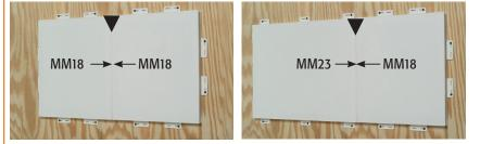
Seal joint channel with Arlington's DSC1 duct sealing compound. See page S-11.
