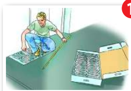
Lay out Reflect Plates
