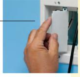
Note Install voltage separator for power and low voltage.
