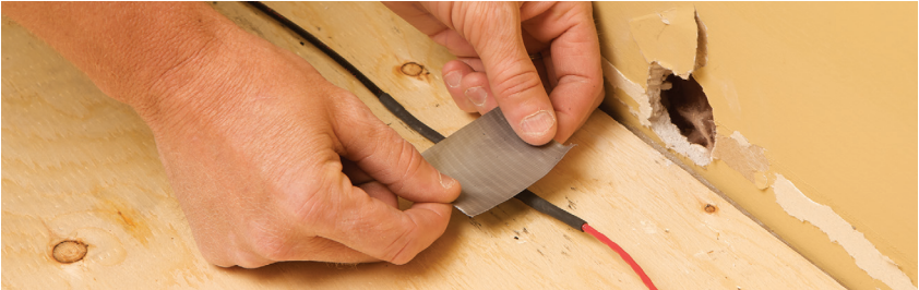
FIGURE 2.23: Secure the cold lead to the subfloor
