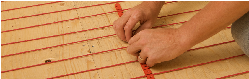
FIGURE 2.29: Install stabilizing guides
