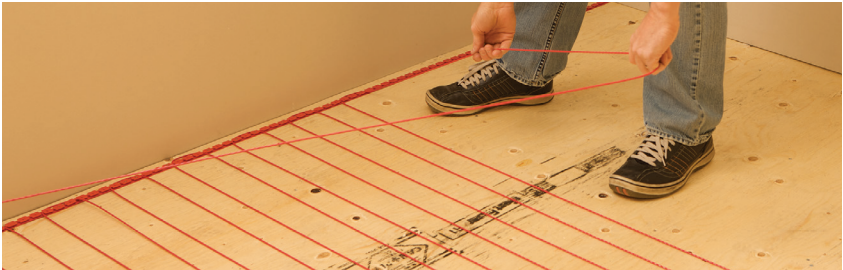
FIGURE 2.27: Install the heating cable
