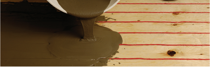
FIGURE 2.42: Self-leveling compound method
