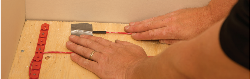
FIGURE 2.28: Secure the end seal
