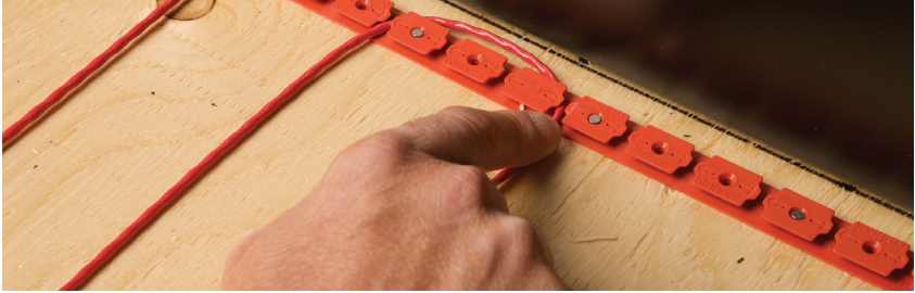
FIGURE 2.26: Install the heating cable
