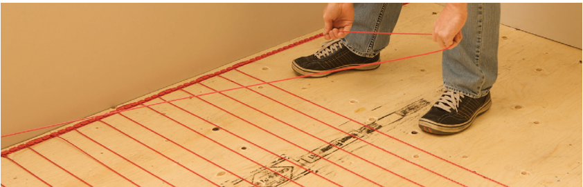
FIGURE 2.27 : Installer le câble chauffant
